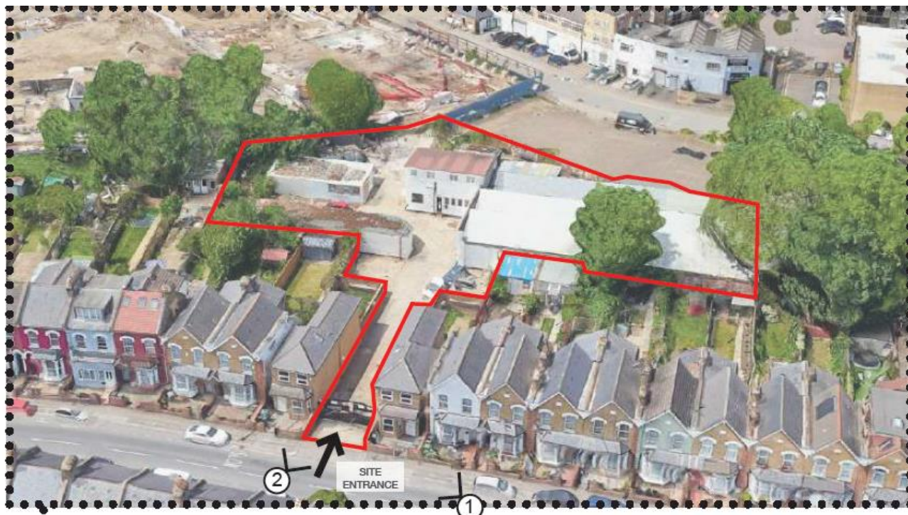
Fig 1: site location in context
