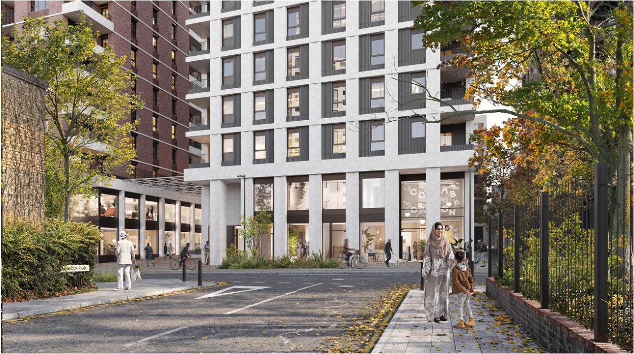
Clarendon Road Approach View
